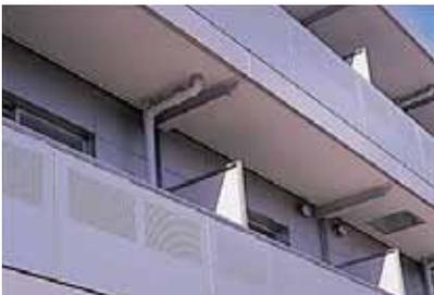
Blind panel under balcony handrail, partially perforated panels, Japan
