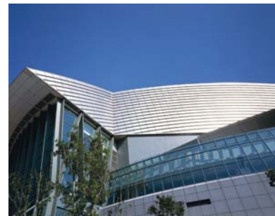
Taipei Arena, Taipei, Taiwan TCM is used for the external cladding underneath the roof.
